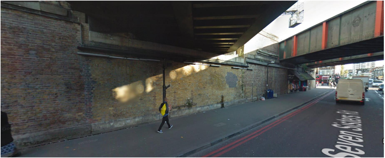
Image 2: View of northern abutments under bridges
